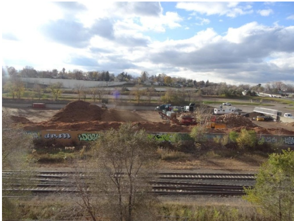
Parcel 6 from elevator tower, Parcel 7 beyond
