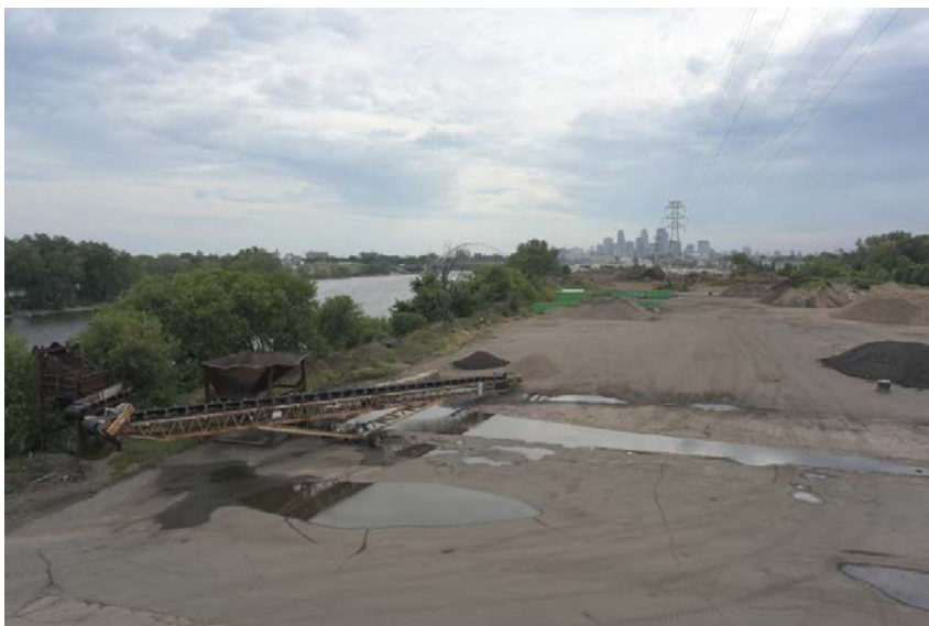
Looking south/downriver from warehouse roof towards Parcels 3 -- 5
