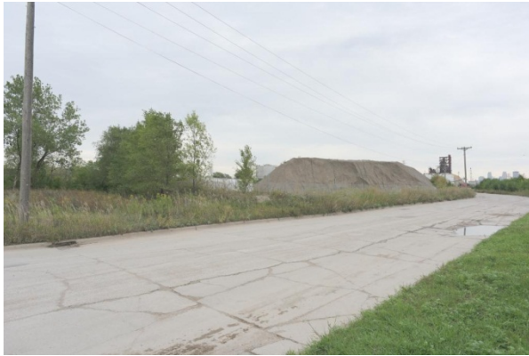
Parcel 1 from northern end; First St. N. in foreground and extending downriver (south) towards Dowling
