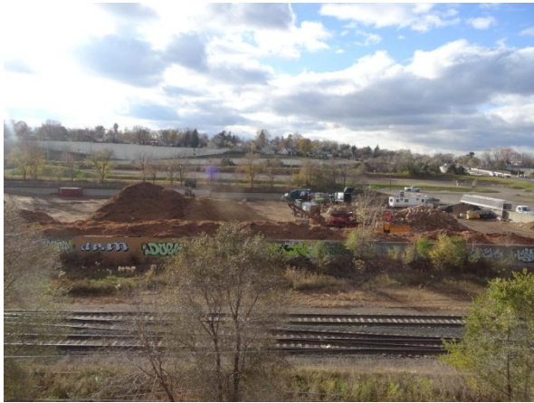
Parcel 6 from elevator tower, Parcel 7 beyond
